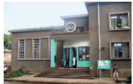
3. Entrance of the NALE old building.
