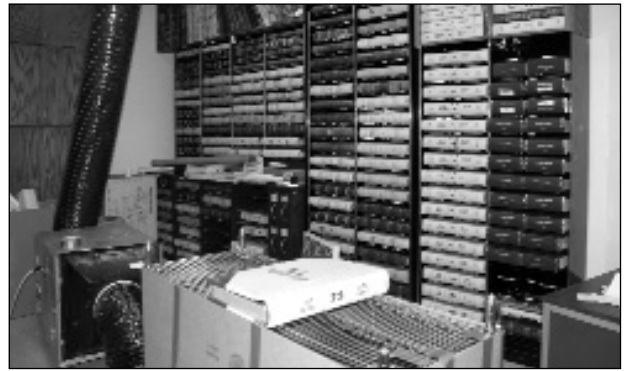
Record book storage vault with metal roller shelving; a temporary positive air ventilation system is set up to help with soot extraction.
