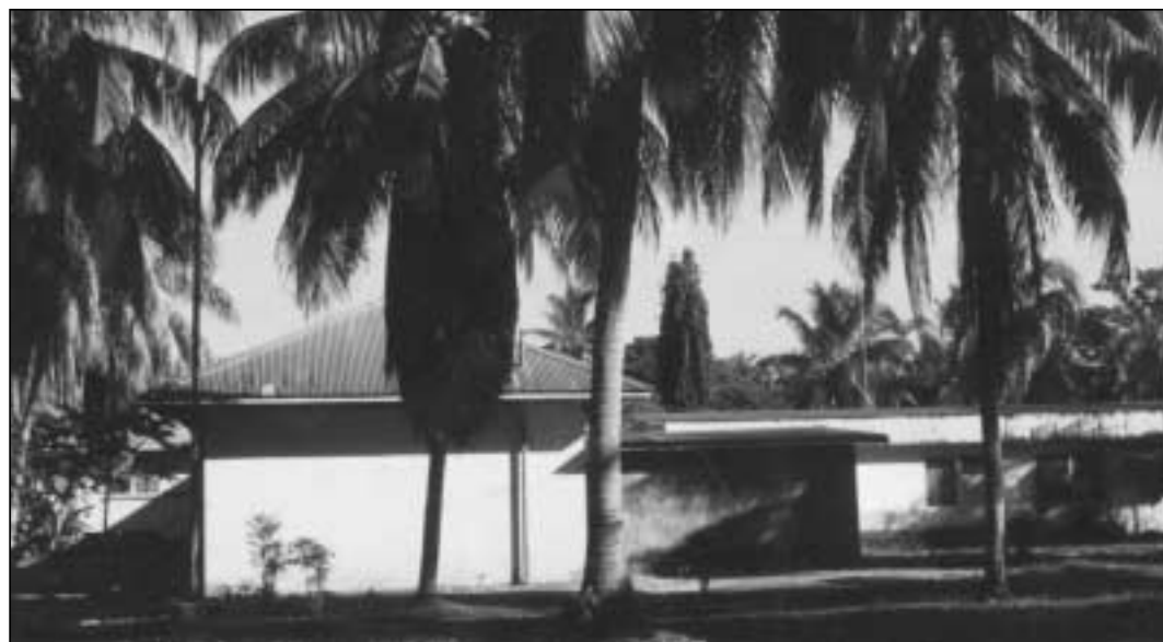
Archives repository and administration block. Russell Islands Plantations Estates Ltd, Yandina, Russell Islands, Solomon Islands.
