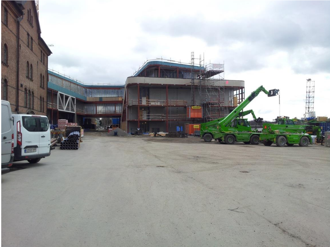
The building site
