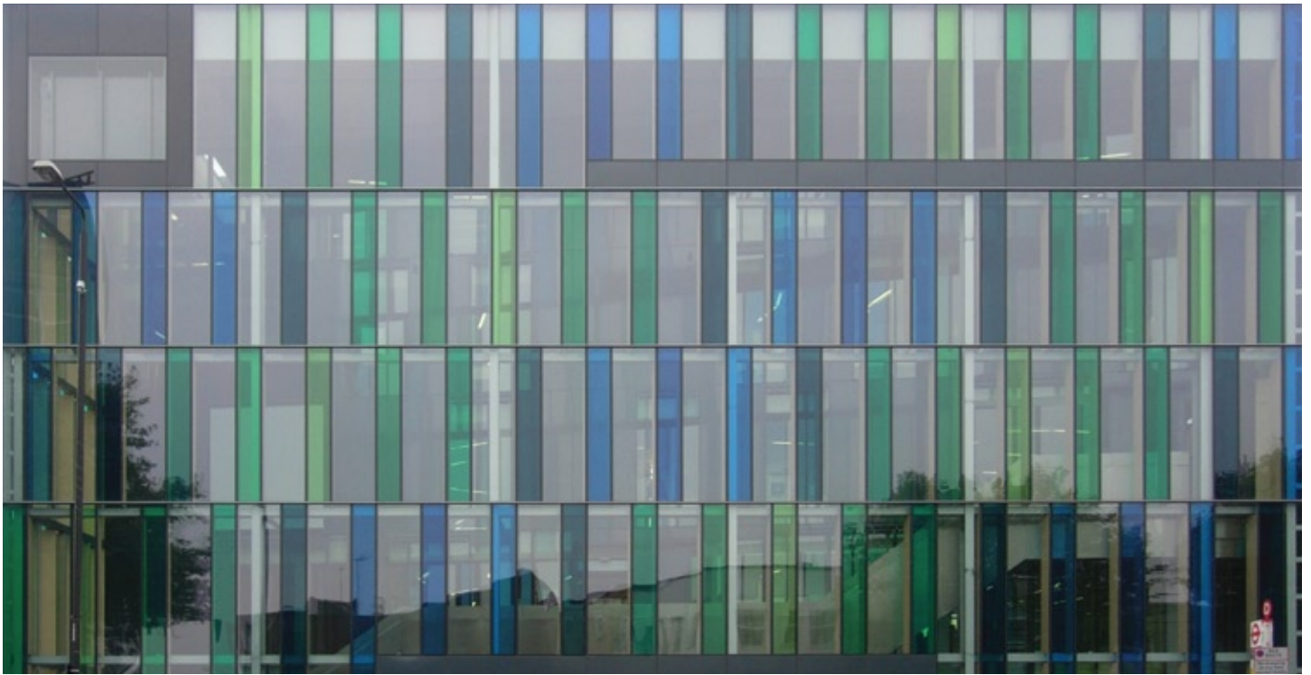
THE LIBRARY WILL BE AN OPEN LEARNING SPACE: Idea Store Whitechapel, London, United Kingdom; outside view, architect: David Adjaye.
